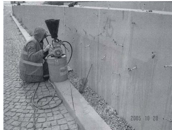
Figure 4. Grouting of low-quality concrete
