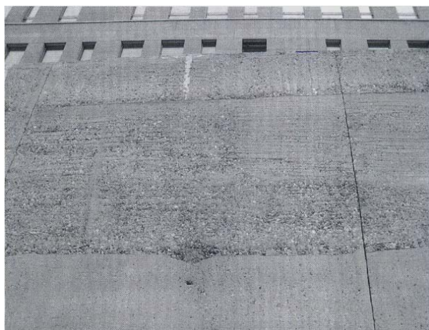
Figure 3. Low-quality waterproof concrete
