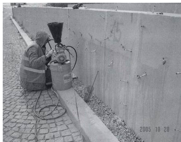
Figure 4. Grouting of low-quality concrete
