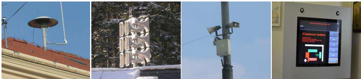
Figure 1 - 4 Currently used end warning elements in the Czech Republic – rotary siren, electronic siren, local information system and information panel (Note: Figure 1 - 3 own), (Náčvik, 2023)
