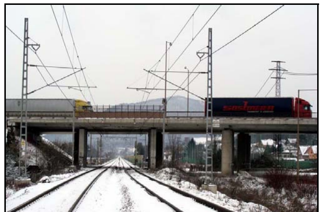
Figure 7. Grade – separated railway crossing.
