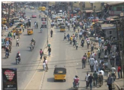
Figure 10. A section of road in Ikeja
