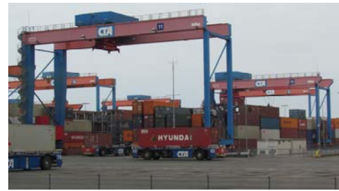
Figure 2. Rail-mounted gantry cranes in the Container Terminal Altenwerder in the port of Hamburg, source: author
