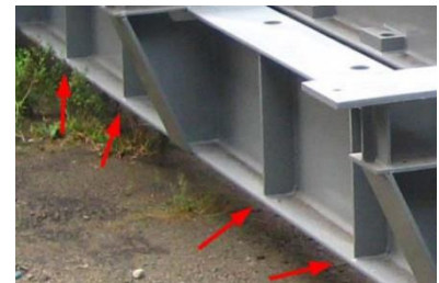
Figure 10: Detail of the numerical simulation of the steel column collapse with additional ribbing (left) and additional ribs on steel H-profile building structure beam (right). Source: Authors.
